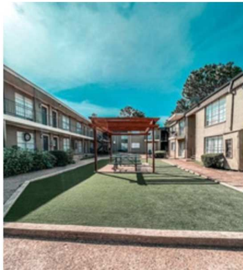
Vista Del Lago Apartments Dallas, TX Units: 320 Purchase Price: $30,000,000 Status: Ongoing Project
